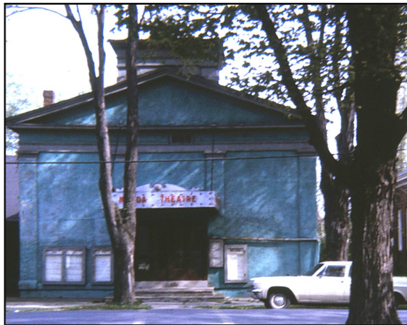
This image was taken after the Nunda Theatre closed in the 1960s. The popular movie house was once the first Church of the Redeemer. Although it was heavily renovated over the years, the Greek Revival lines of the original church were still visible.
